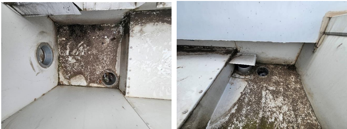
Non-compliant sumps and overflows
